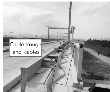
Figure 1.3 Cable Trough Laying of a High-speed Railway
