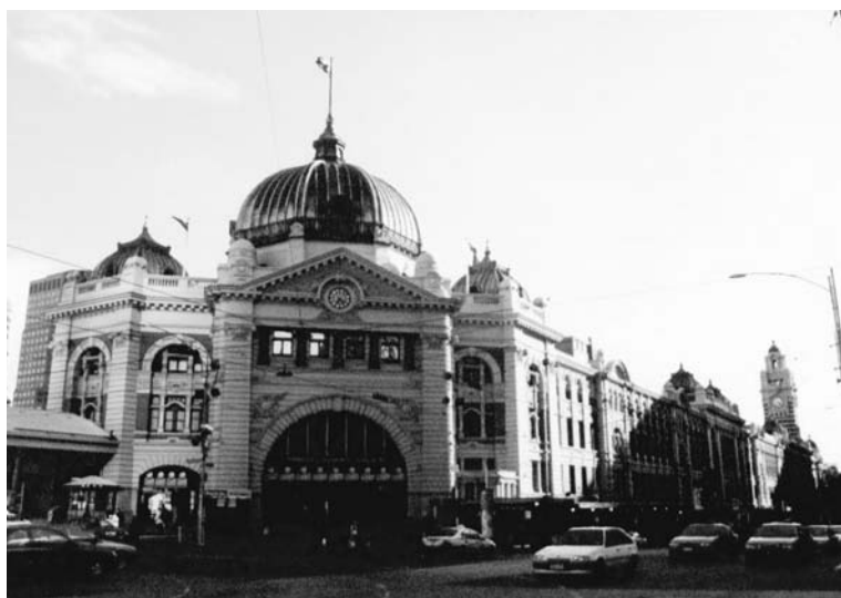
The Flinders Railway Station, Melbourne
