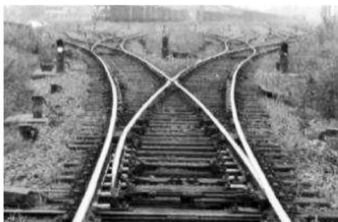
Fig. 1-14 Symmetrical turnout
