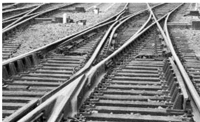
Fig. 1-15 Dual-gauge slip switch turnout
